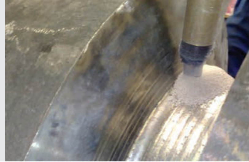
Sub arc welding of Alloy 625
